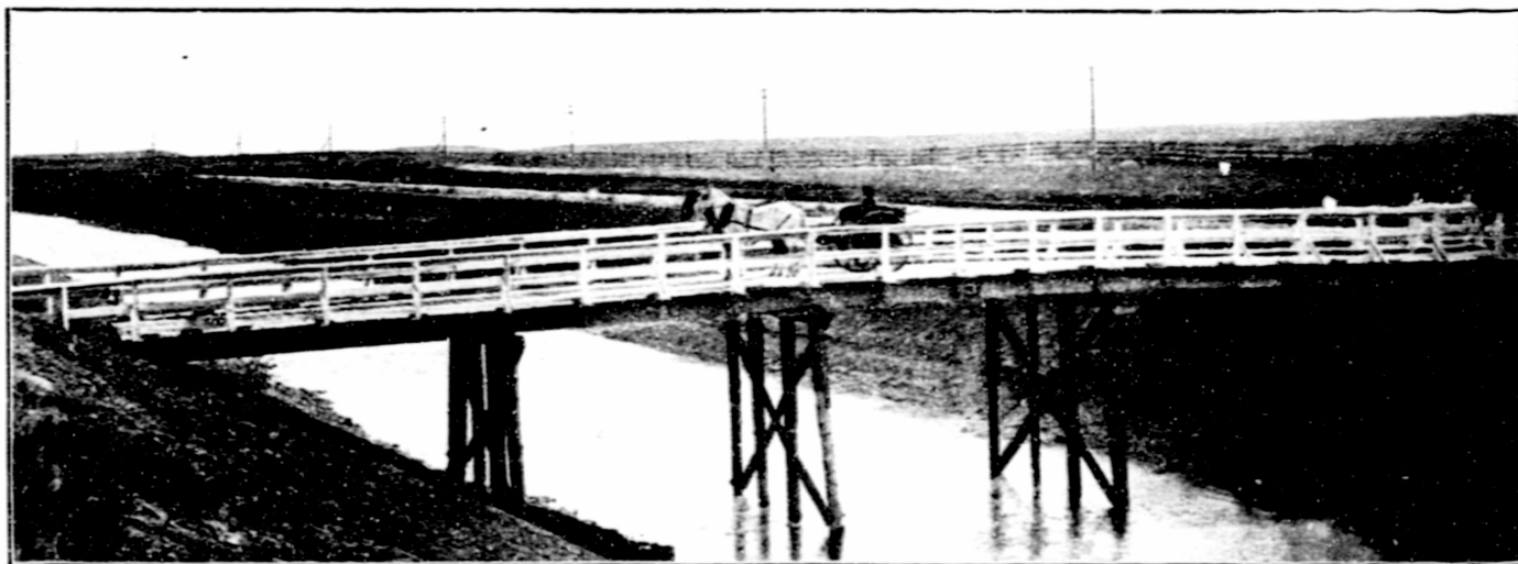
Traffic Bridge over an Irrigation Canal
