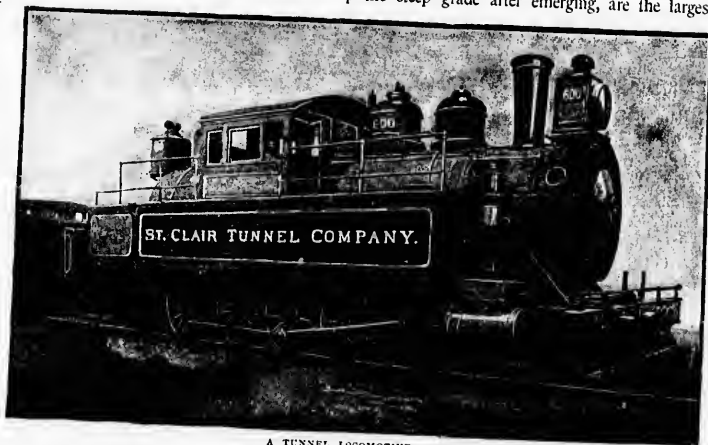
A TUNNEL LOCOMOTIVE.
