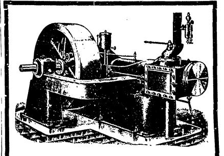
The out-board bearing on the Robb-Armstrong Engine, up to 100 horse power, is connected to the bed by a wing as shown in cut, keeping the bearing perfectly in line. This is a great advantage, particularly for portable saw-mill purposes.
