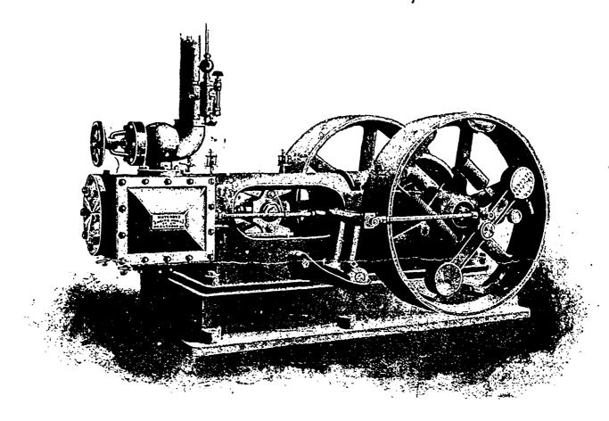
Perfect Balance—photographs of 50 h.p. placed on rollers, not held down by bolts or other wise, running at full speed, show Engine clear cut and still except in reciprocating parts.
