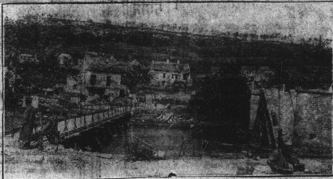
WHERE THE AMERICANS HAD TO CROSS A STREAM The Bridges at Bazoches, in France, as the first of the Pershing Forces Entered the Place.
