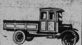
Platform express body with weather-proof cab for cartage, express, wholesalers and general delivery.
