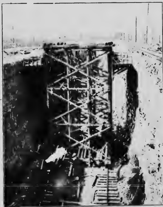
FIG. 4—SCALING TOWER IN ROCK CUT NEAR FOREBAY
