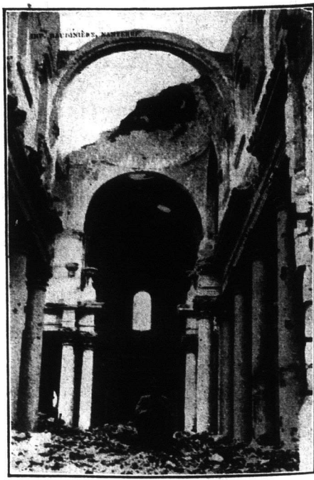
A portion of the cathedral, showing the damage done after a bombardment.
