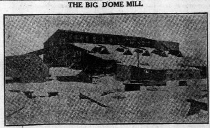
Mill now has the largest capacity in Porcupine district. The tube mill is running 1200 tons a day, and the stamps 1000 tons. Another tube mill of same capacity will be running by March. It is possible the stamps will then be discarded.
