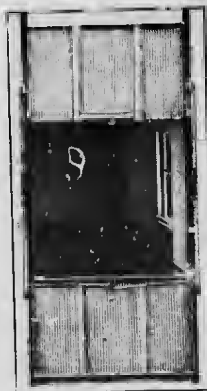
VAMANCO DOOR IN OPEN POSITION, SHAFT SIDE.
