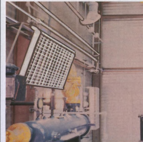
CIS-CAN manufactures five models of flameless infrared gas heaters for industrial heating applications in hazardous areas.
