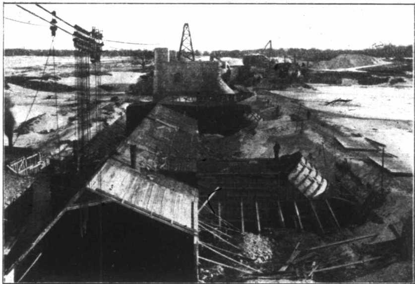
Construction of Dam during Winter, St. Andrews Locks, Red River.
