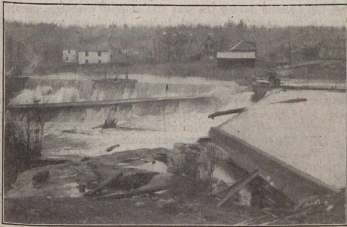
FIG. 7—VIEW ACROSS OLD POWER DAM, SHOWING HEADWATER AT RIGHT AND LOG CHUTE
