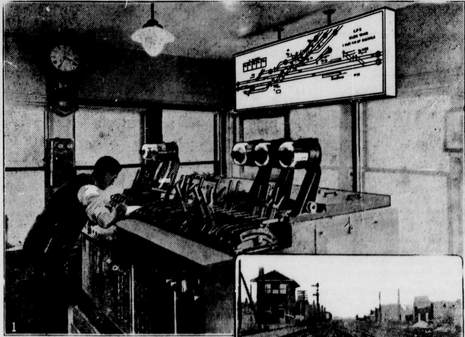
Above.—Interior of the Canadian Pacific Westmount Interlocking tower, showing the control levers and the illuminated plan, the light bulbs appearing as black spots.
