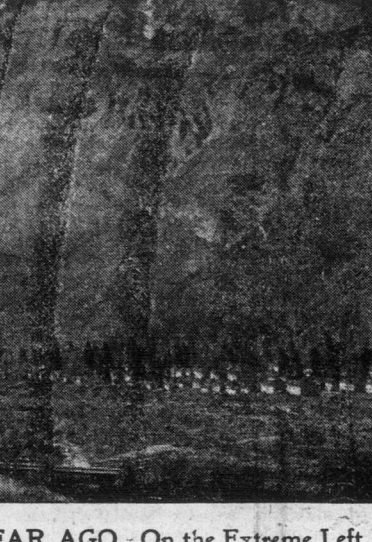
VIEW OF FRANK COAL MINE FRANK ALBERTA
