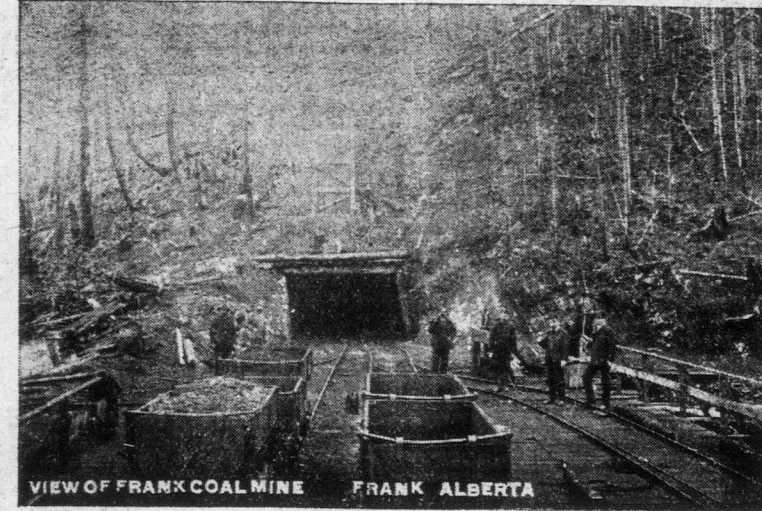
MAIN ENTRY OF COAL MINE—Showing Tunnel to the property of the Canadian American Coal and Coke Co., Frank.
