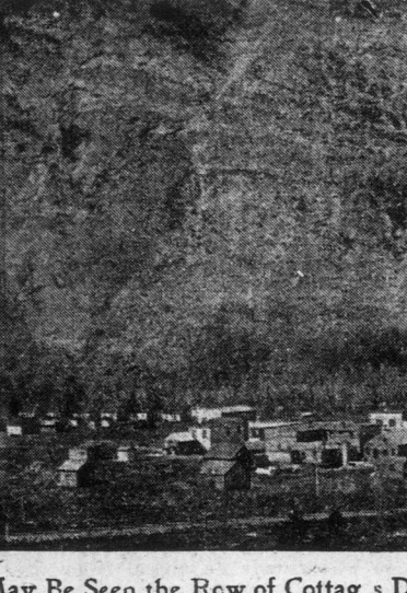
TOWN OF FRANK A YEAR AGO - On the Extreme Left May Be Seen the Row of Cottages Destroyed by the Landslide
