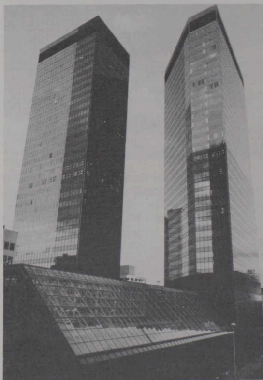
Toronto-Dominion Square in Calgary's Home Oil Tower.
