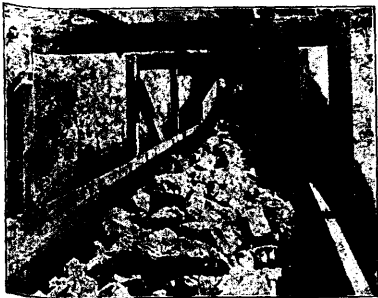
Conveyor 328 feet centers, handling 4 tons "run of mine" coal per minute.
