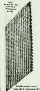
NO DARK BUILDINGS, rooms, or basements where this glass is used. CIVES 5 TO 40% MORE LIGHT than any flat-back prismatic glass on the market. ORNAMENTAL IN APPEARANCE inside and out. STRENCTH immeasurably increased. Does not crack like ordinary prismatic glass DIFFUSION OF LIGHT is complete. ALL SHADOWS ELIMINATED.
