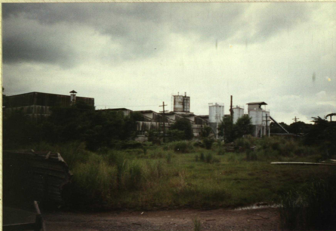
No. 23. Distant view of lightweight concrete plant.
