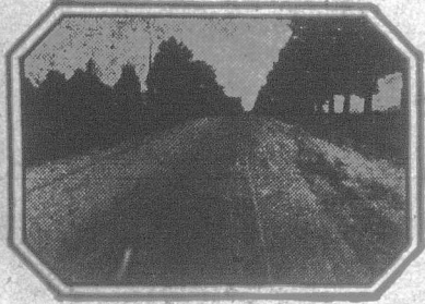
After same road was built with Tarvia Filled Macadam
