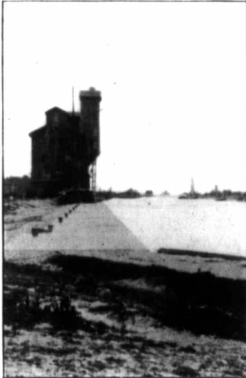
East Wall, Inner Harbor, Port Colborne, Ont. Hogon & Macdonell Contractors
