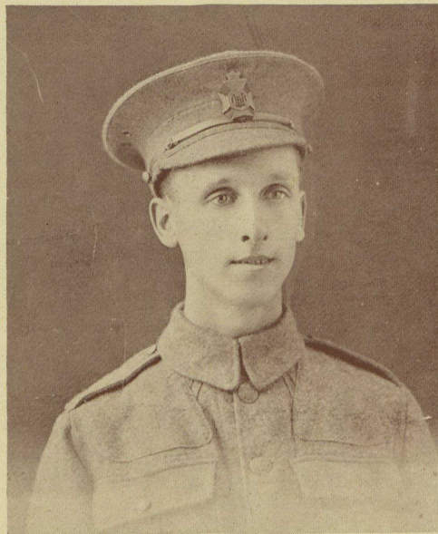
Rifleman Richard Newberry (London Staff) of the Queen's Westminster Rifles, was killed on March 28th, 1918, before Arras. Mr. Newberry's connection with the Company dates back to 1903. He was at first attached to the Counting House, but later was put in charge of the Spares Order and Invoicing Department. He joined the Colors in March, 1917, and within three months was in France. He was married and leaves a widow and young son.
