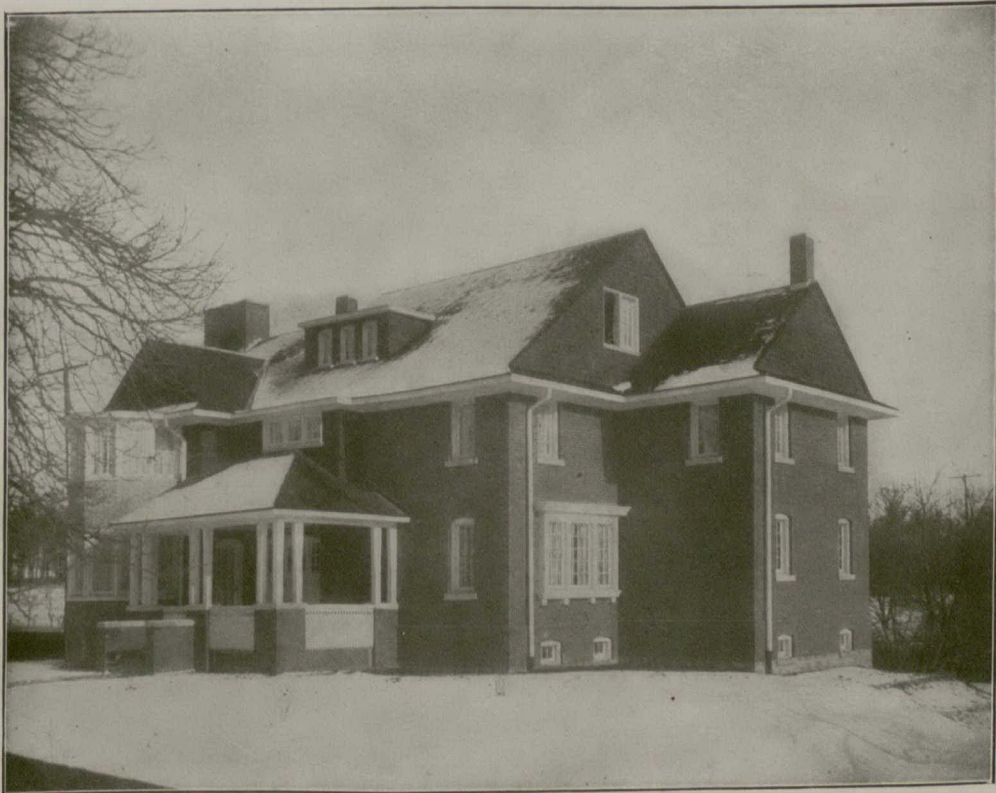
VIEW OF HOUSE SPACE FROM SOUTH-EAST.
