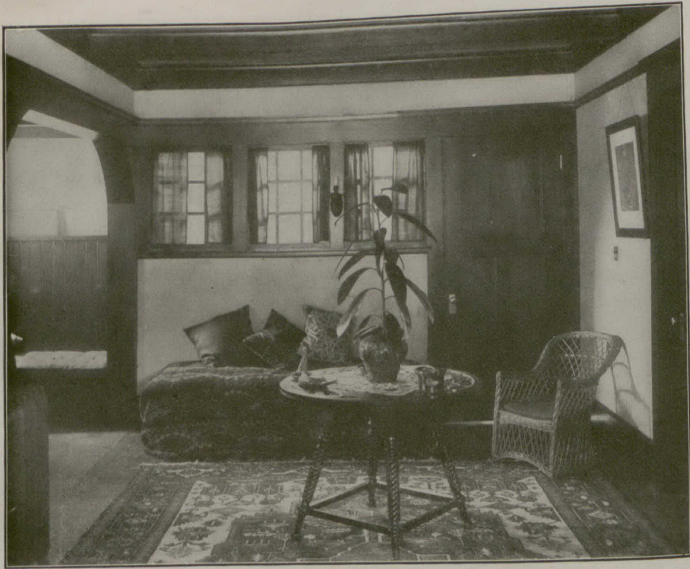
VIEW OF NORTH END OF HALL, GROUND FLOOR.
