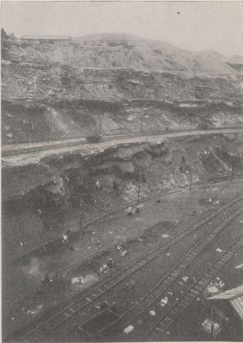
Fig. 25 shows one of the open-cut coal-mines in Fushun
