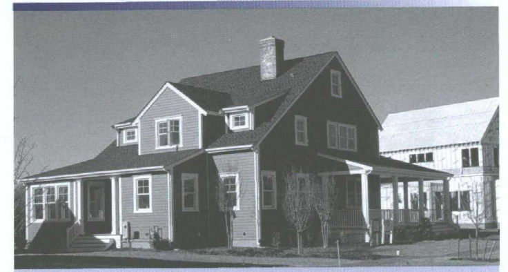
A DAC International home in Easton, Maryland.
