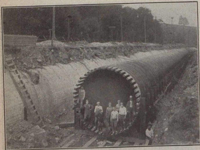
NO. 3 CONDUIT, SHOWING MUDSILLS IN POSITION—NO. 2 CONCRETE CONDUIT EXPOSED
