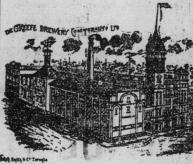
The refrigerating plant referred to in former notice is now fully completed, egether with the water tower, gradework, together with the water tower, gradework, attemperators, refrigerators, etc., etc. all operated by the De La Vergue System, which is working admirably.
