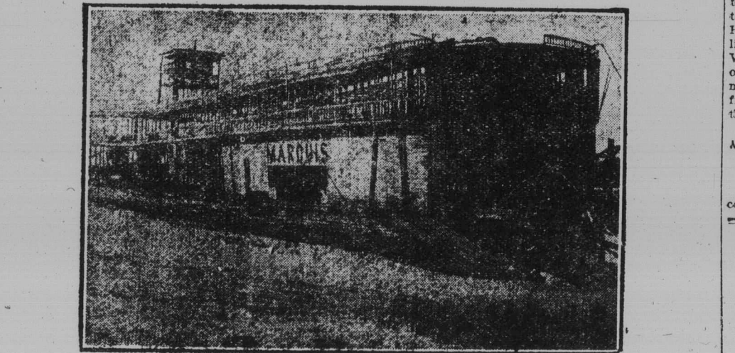
Rotted timbers on the banks of the North Saskatchewan river at Prince Albert are all that is left of the old stern-wheeler Marquis, which once plied between Cumberland House, Sask., and Edmonton, Alta.
