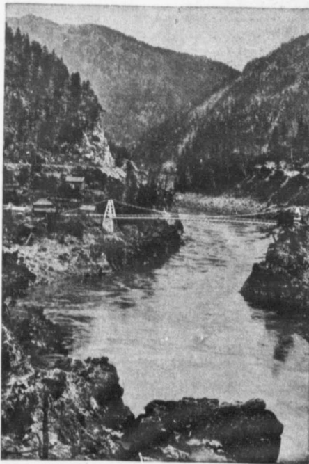
CARIBOO ROAD BRIDGE.
