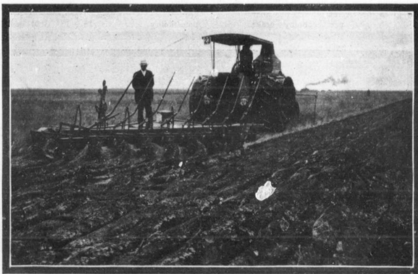
The Rumely 30-60 Oil-Pull Tractor pulling an Eight Bottom Engine Gang. (Gold medal winner Class E)
