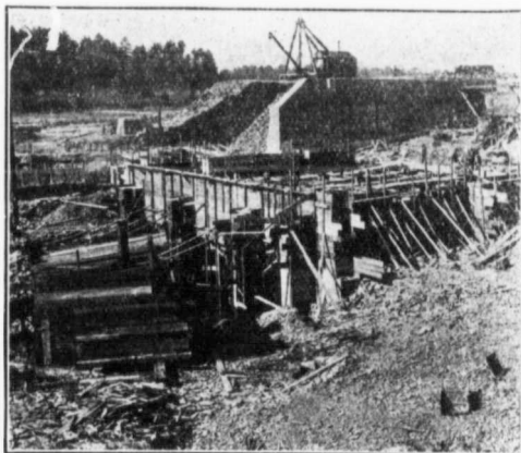
Fig. 3—General View of Power House, Floor Level.
