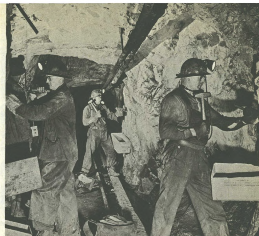
Hard-rock miners chip samples off a drift at the 1900-ft. level.
