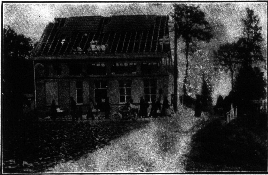
Refugees Leaving Steenstraate Bridge before the Big German Onslaught It was at Steenstraate Bridge that the Germans succeeded in getting over the Yser and established a bridgehead. Later, however, the Allies drove them back across the river. The house seen in the photo was converted into a veritable fortress.
