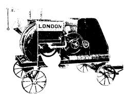
A portable machine made in two sizes, suitable for small jobs, such as building foundations, sidewalks, barn walls, concrete sites or any work requiring a capacity up to 60 cm. yds. per day.
