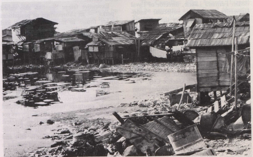
In Asia's cities, squatter settlements are swelling rapidly creating massive needs for shelter, employment, clean water and other services.
