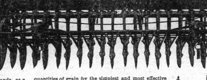
quantities of grain by the simplest and most effective feed construction known. Another feature of McCormick Drills is the bearings. They are as nearly dust-proof as it is possible for drill bearings to be. Only clean oil reaches the cones, keeping the bearings running smoothly and without friction.
