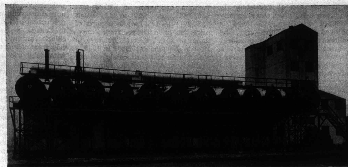
Refinery for Coal Tar Chemicals Erected in Toronto in 1931. New plant of Dominion Tar & Chemical Company Limited, in which pure phenol is manufactured for the Canadian market. This is a product which was formerly imported. In addition, creosols and other tar acids are produced.
