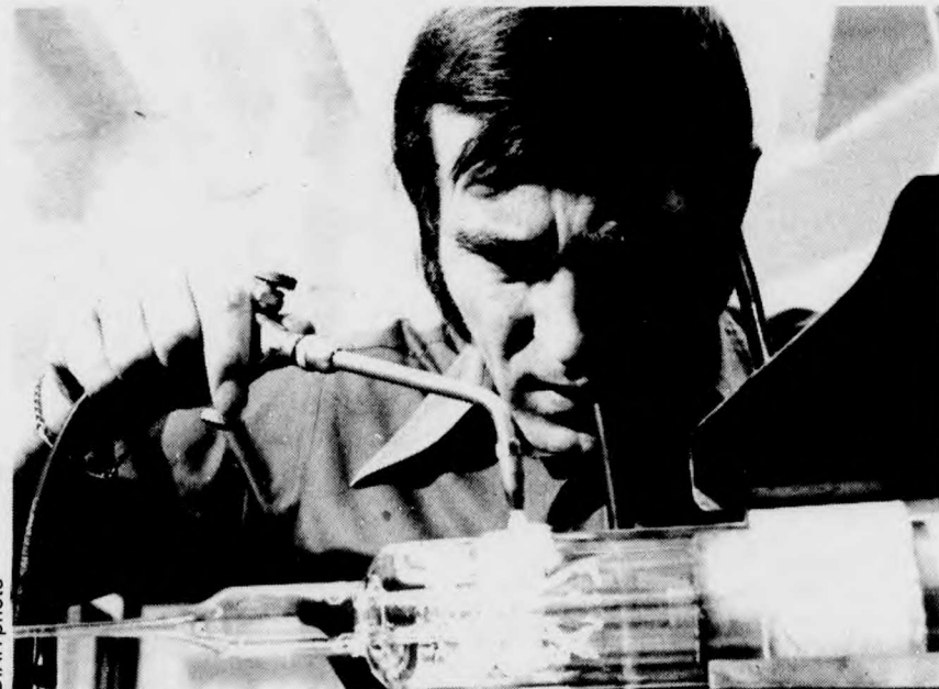
Ed Verdoold creates a Mercury Diffusion Pump.
