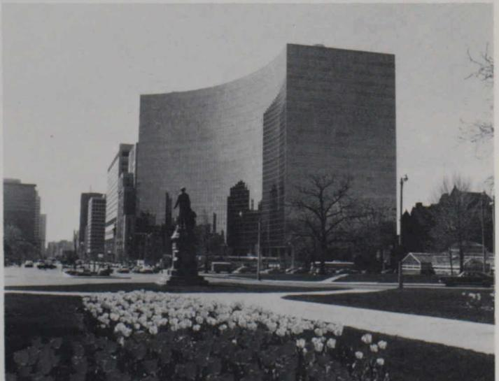
Hydro Place, which has no furnace, recently came through the coldest Toronto winter in forty-three years with heat to spare. The energy system is not solar; the outer "skin" of the building is designed to exclude as much solar heat as possible.
