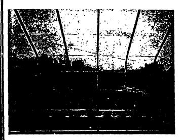
The Eave Line is Where The Ordinary House Rots Out, Because The Condensation Gets into the Joints: The U-Bar House Has No Eave Joints. It is The Original Curved Eave House.
