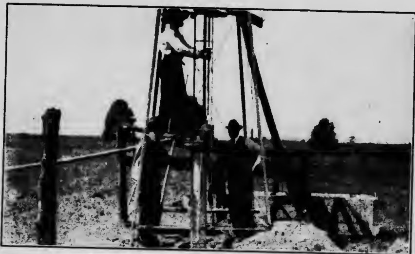
Fig. 5.—(a) Sinking the open 10-inch drive pipe.
