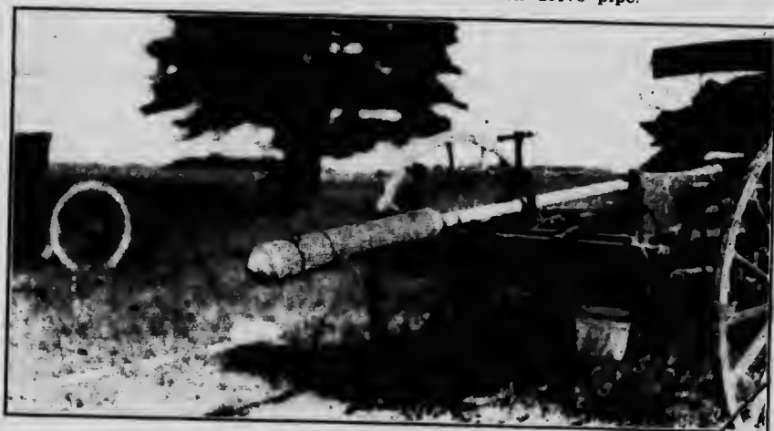
Fig. 5.—(b) Sand filter, to be placed in open drive pipe.
