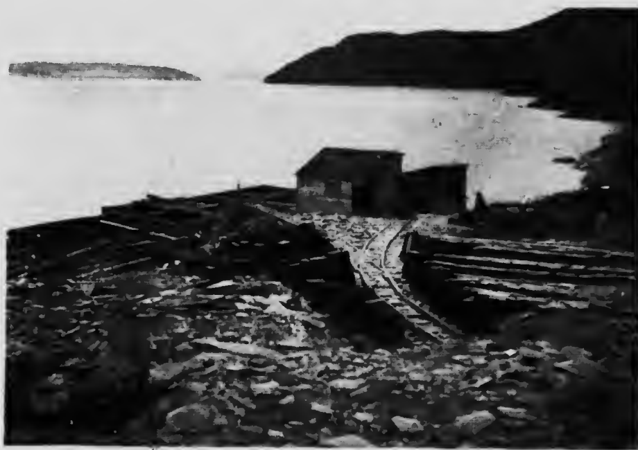
A VIEW OF SMITH SOUND QUARRY, NEWFOUNDLAND.
