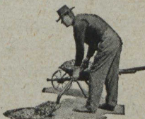
The mixture of "Tarvia-KP," stone and sand, is placed in the prepared hole.
