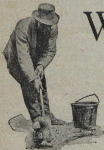
The hole to be patched is cleaned and the bottom and sides are painted with "Tarvia-KP."
