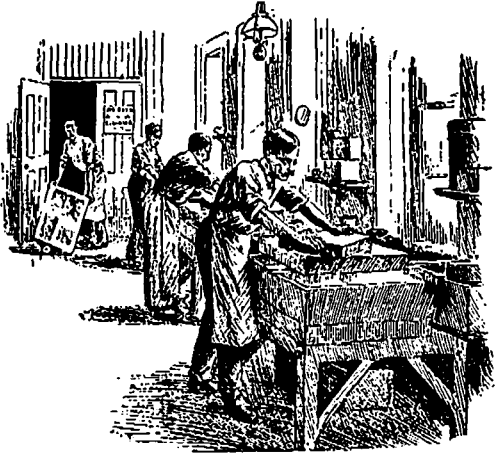
PREPARING THE STONES.
