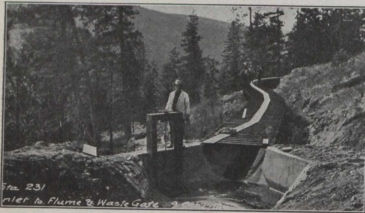
Inlet to Flume and Waste Gate.
