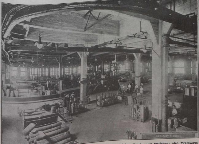
Fig. 11.—General View of M., K. & T. Terminal at St. Louis, Showing Telpher Tracks and Switches; also Tramways Platforms and Hatchways.
