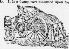
wheels. The weight is well distributed on both front and rear wheels, thus avoiding either upward or downward pressure on the team. The tilting of the cart is effected by a crank and gear mechanism in connection with a rack and pinion, which not only renders easy the tilting of a heavy load, but is also of great advantage when it is desired to load the cart with shovel, as the cart can be firmly held in any position from level to completely dumped.
