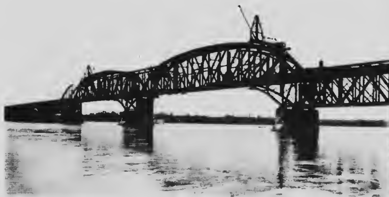
1st and 2nd 408 foot spans ready to launch Dismantling old channel spans
