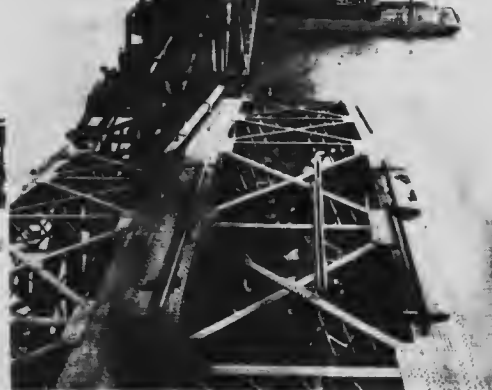
10th 408 foot span ready to launch
