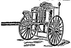
This machine is the most powerful are ngater. It has two cymicers, to get with which it comes in contact non-inflammable, and will not corrode when not in use. For full the Head Office of the Company at Kingston. his machine is the most powerful fire fighter. It has two cylinders, 40 gallons capacity particulars, write to the Head Office of the Company at Kingston.
