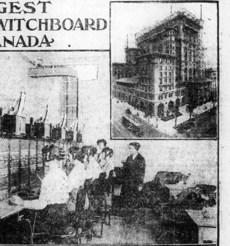
The Maids' Signal Service helps the guests to find maids when required. On the telephone switchboard are hundreds of small lamps bearing numbers corresponding to the numbers of the guest rooms. Each maid is provided with a miniature portable lamp, and before entering a guest room, she places this lamp in a socket on the outside door trim of the particular room. Immediately after being placed in the socket the lamp lights, and anybody passing can know that there is a maid in any room whose door is illuminated by a lamp. The placing of the maids' lamp in the socket also causes a lamp bearing a similar number stationed on the telephone switchboard to light, thereby notifying the telephone operator of the room in which a maid is engaged. From the lamps on the switchboard the operator knows where all the maids are to be found, and should a guest require the attendance of one she can be immediately summoned by telephone message.
